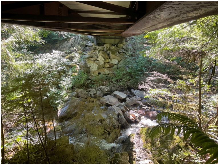
Right Bank Abutment when facing downstream
