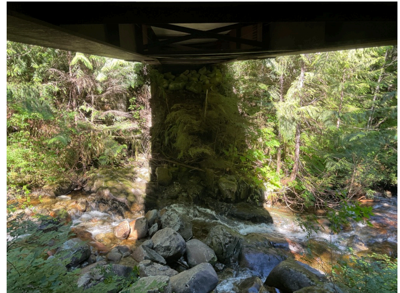
Left Bank Abutment when facing downstream
